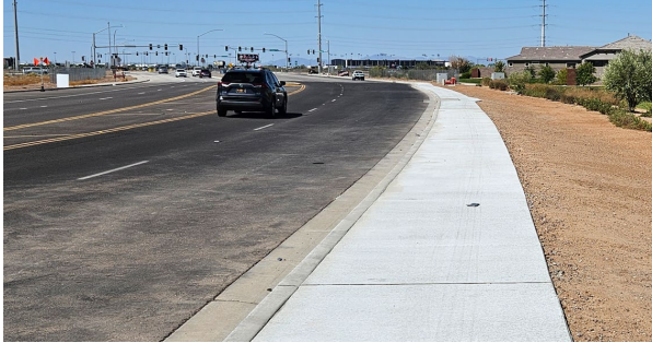
Williams Field Rd Sidewalk Installation
