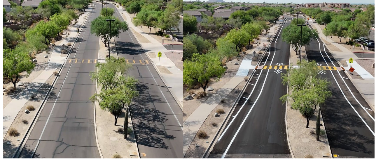
Las Sendas Elementary Raised Crosswalks
